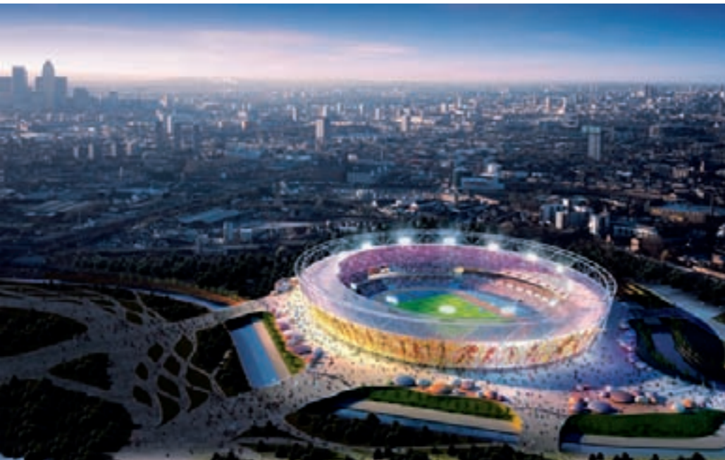
ACO SPORT elements in London. ACO has provided drainage systems for all the Olympic stadiums since the Olympic Games in Munich 1972, with the exception of Moscow
