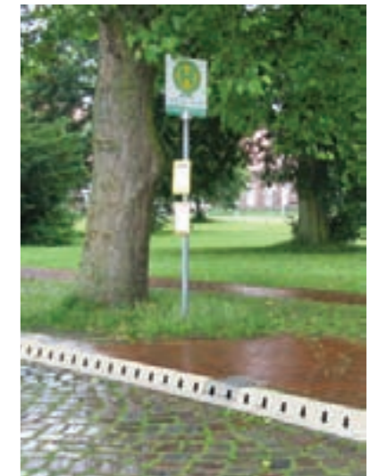
Kerbstone and drain in one, ACO DRAIN® KerbDrain
