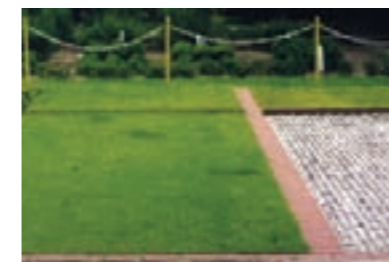
Parking space reinforced with grass grid
