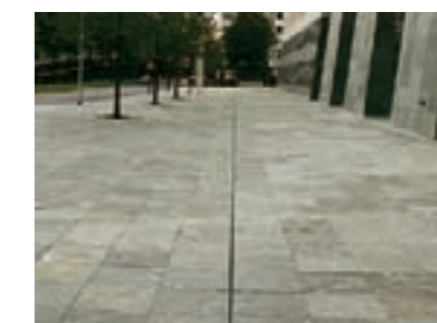
Slotted channels for abutting paving stones are harmoniously integrated into the overall floor surface. These can be custom manufactured, individually with or without an integrated gradient, in straight, radial or polygonal designs
