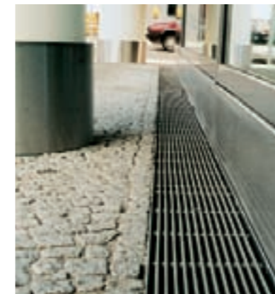
Channel drains in stainless steel combined with a wide range of different grating types, provide design accents as well as safely draining away water from façades and paved surfaces
